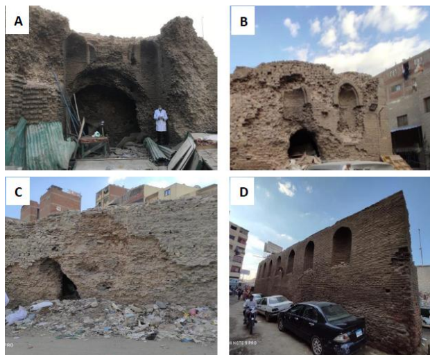
Fig. 1. The four façades of the intake tower of the Ahmed IbnTulun Aqueduct: (A) Eastern (main) façade; (B) Western façade; (C) Northern façade; (D) Southern façade. (Photographs taken by the authors).
