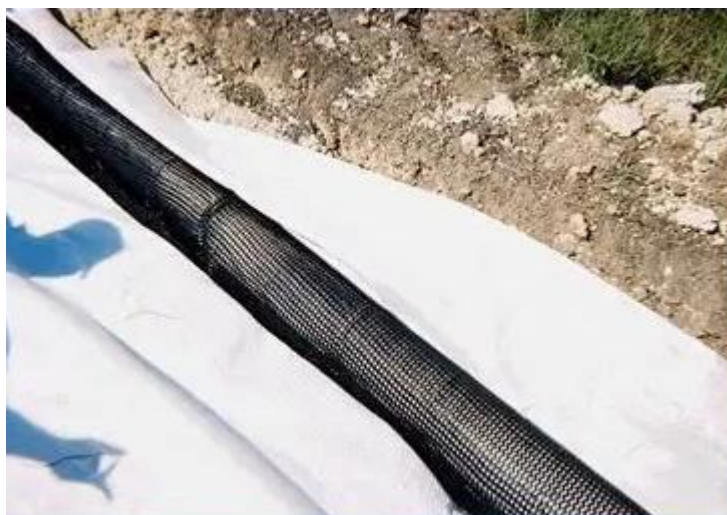
Figure 5. Subsurface drainage by geotextiles.
