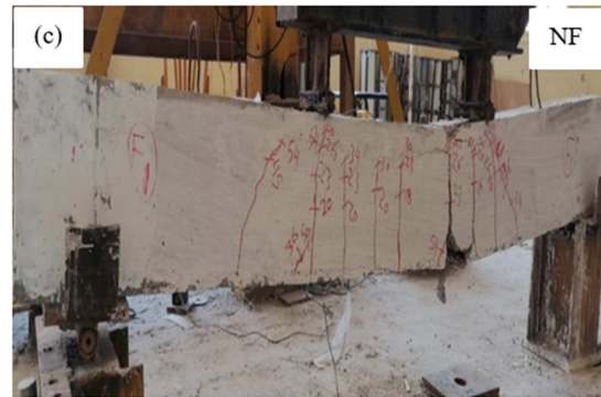
Figure 16: Crack patterns and failure shapes of normal concrete with GFRP
