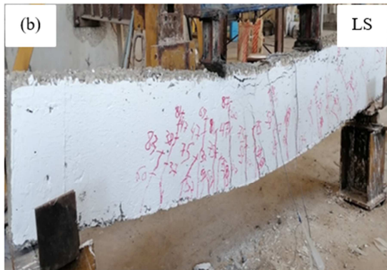
Figure 15: Crack patterns and failure shapes of lightweight concrete with steel reinforcement
