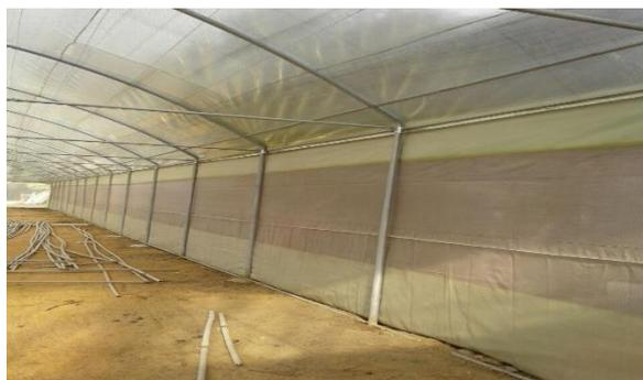
**Figure (5):** Inside columns structure of the greenhouse
